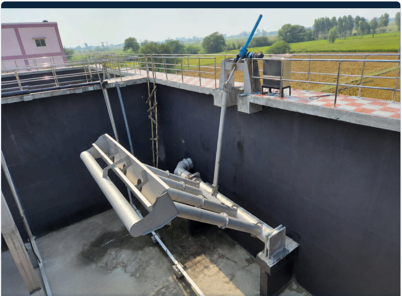
🔧 Floating Assembly with Flexible Swivel Joints & Motorized Control[cite: 1]
